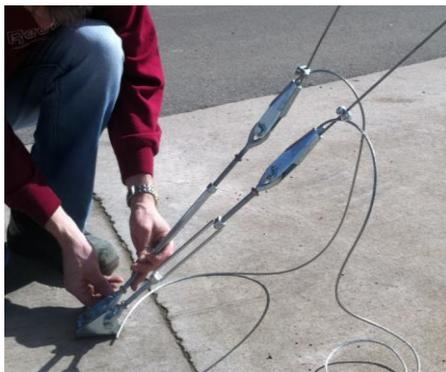
The length of the guy-ropes can be adjusted by feeding through the wedge socket so that most of the tension is applied prior to making any adjustment to the turnbuckle ends. Tighten the rope grips.
