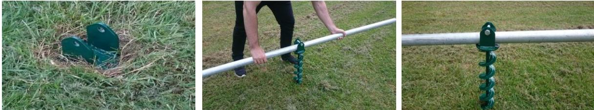
Various obstacles such as; tree roots, bricks or stones can be encountered and are usually easily overcome using a piece of pipe or scaffolding for greater leverage through the anchor head. Ensure that the anchor is perpendicular to the ground beneath for minimal disturbance to the soil and best anchoring effect.
