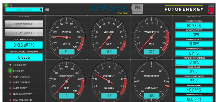
AirForce ® control web portal
